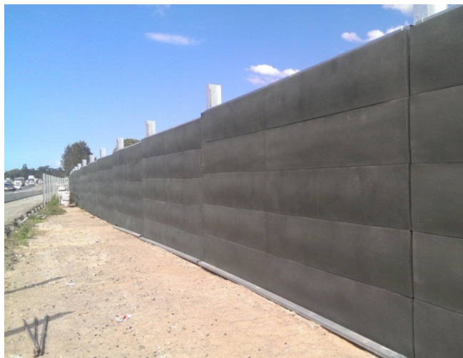
Installed panels at Noisewall 2W03
